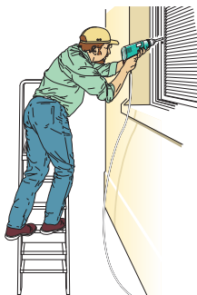
Figure 2a Incorrect - steps side-on to work activity
